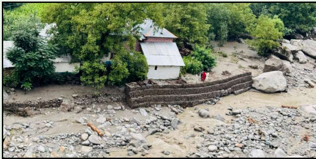
UC Kundal Shahi, Village Satra 01 Gabion Wall, Length 120 Feet
