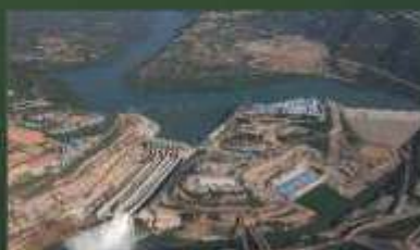
720MW Karot Hydropower Project, AJK/Punjab Estimated Cost US $1698 Million
