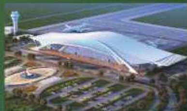
Gwadar International Airport Estimated Cost US $230 Million
