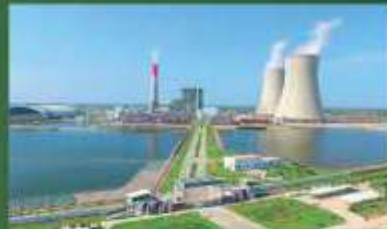
1320MW Sahiwal Coal-fired Power Plant Estimated Cost US $1912 Million
