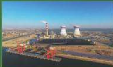
1320MW Coal-fired Power Plant at Port Qasim Karachi Estimated Cost US $1912 Million
