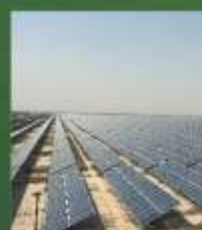
1000MW Quaid-e-Azam Solar Park Bahawalpur Estimated Cost US $1.3 Billion
