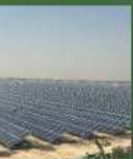
Azam Solar Park Rawalpindi Estimated Cost US $781 Million
