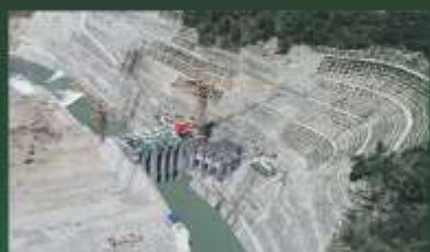
884MW Suki Kinari Hydropower Project, Khyber Pakhtunkhwa Estimated Cost US $1962 Million
