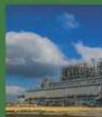
1320MW China Huadian Power Project, Havelian Estimated Cost US $1.3 Billion
