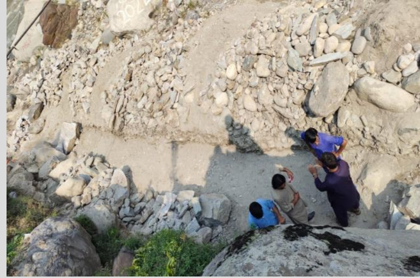
Figure 11 Garan -1 Up Stream-Flood Protection Wall Neelum Valley-PRCS
