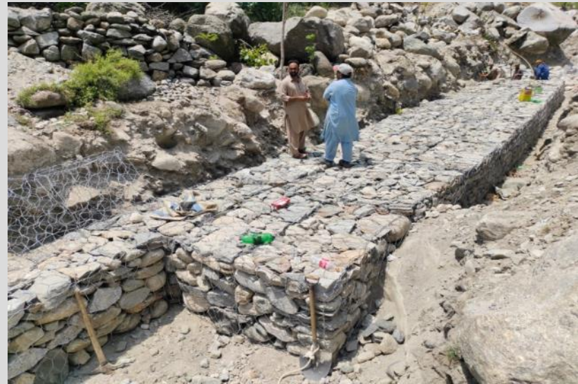
Figure 9: Garan -1 Up Stream-Flood Protection Wall Neelum Valley-PRCS
