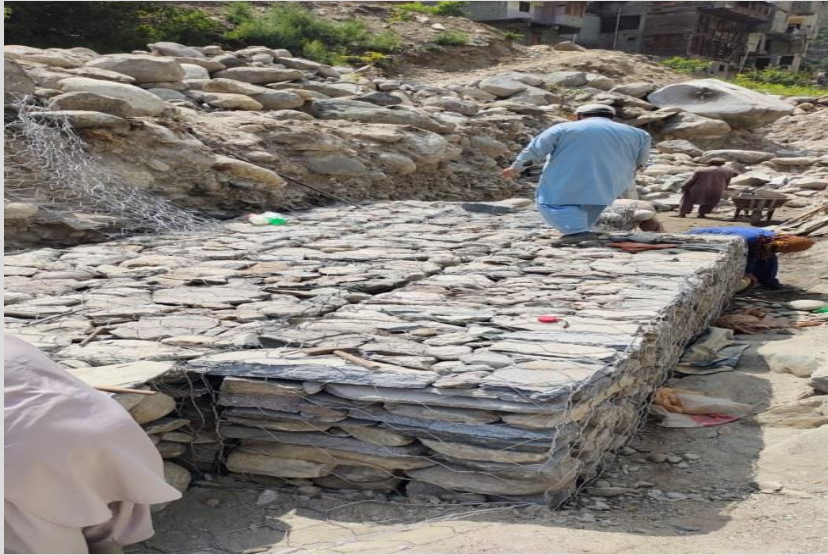
Figure 8: Flood Protection Wall Dullar 1 Neelum Valley-PRCS
