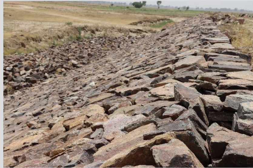
Figure 13: PID Flood Protection Wall in Progress
