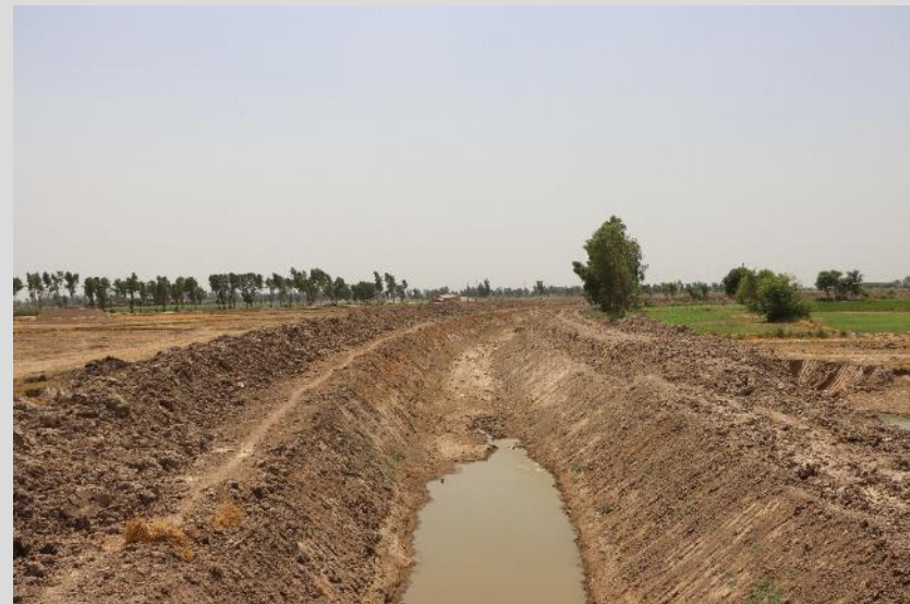
Figure 15: Drain channelization of PID schemes
