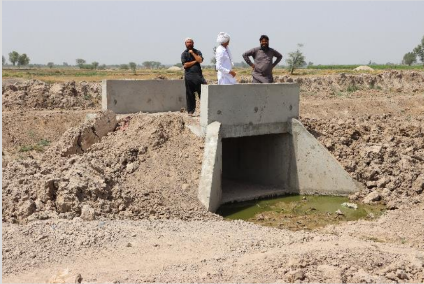
Figure 14: Intake structures in progress on PID schemes
