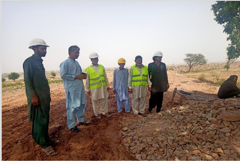
Figure 12: PID Flood Protection Wall PPE Use
