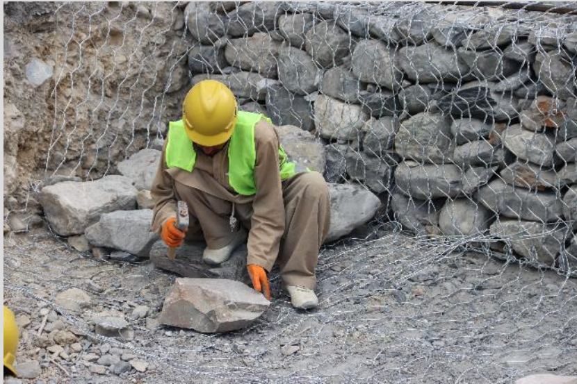
Figure 4: PPE usage in gabion wall construction at Sost Nazimabad
