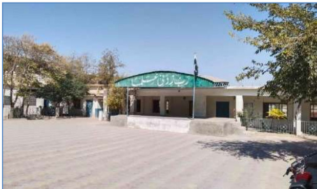
Plate 99: A view of after retrofitting school of Govt. Boys High School at Kechibeg, Siryab Road Quetta.
