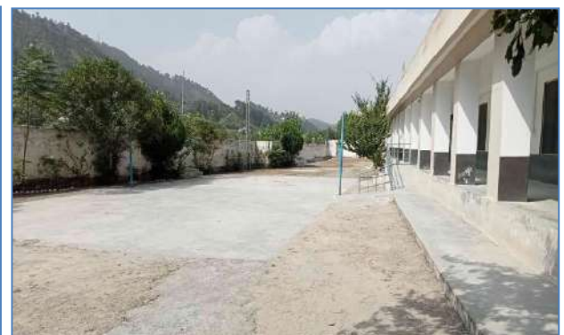
Plate 42: A view of after retrofitting school of GGHS at Dogha, District Mansehra.
