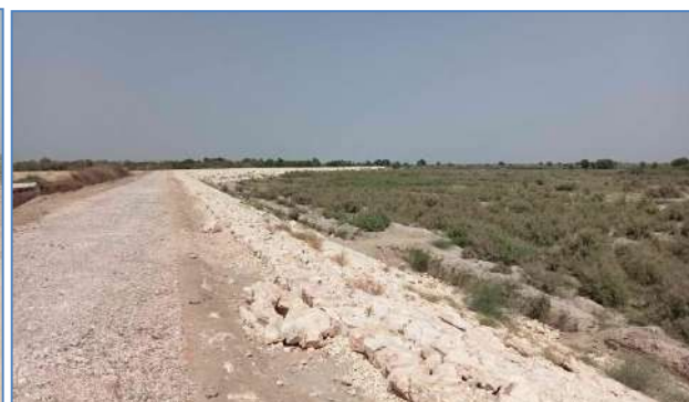
Plate 94: A view of re-constructed stone apron, stone pitching and earth work.
