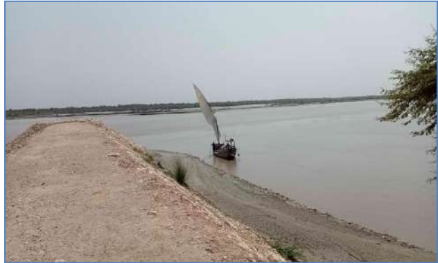
Plate 86: A view of constructed Mole Spurs at Agani Akil village, District Larkana.
