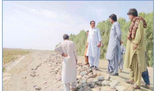
Plate 122: A view of constructed flood protection structure at Killi Muhammad Afzal, Tehsil Dalbandin, District Chaghi.
