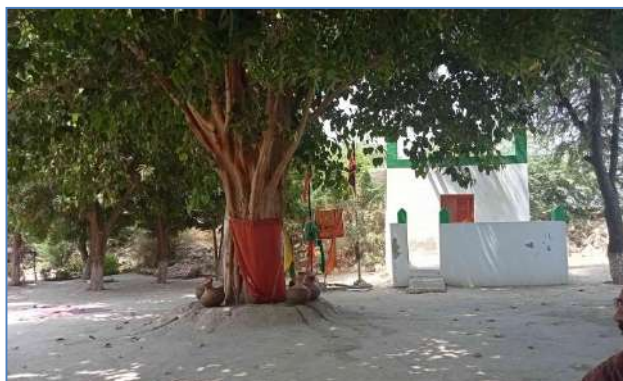
Plate 92: Re-constructed Mole Spurs for protect the Indus river bund and Dargah of Sain Muhammad Shah Khairi which is damaged in flood 2010 at Agani Akil village, District Larkana.
