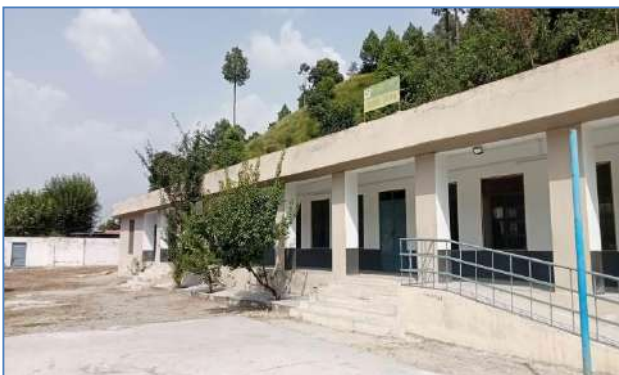
Plate 41: A view of after retrofitting school of GGHS at Dogha, District Mansehra.
