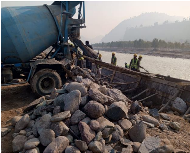
Construction Site & Use of PPEs
