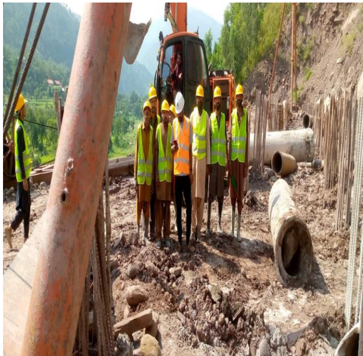
PPE use at AJK Land Slide Project
